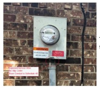
The customer is responsible for installation and maintenance of the meter can and service riser pipe at the house
